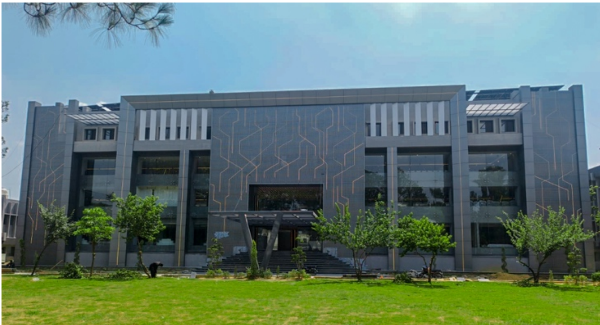
IRADA Head Office main building envelop
